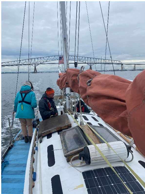
Passing under the Frances Scott Key Bridge. This iconic bridge collapsed March 26, 2024 when struck by containership Dali. RIP six migrant workers! Baltimore Strong!
